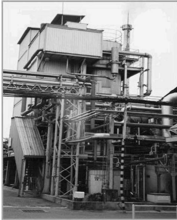
Figure 41 Special boiler using a soy sauce cake. (Courtesy of the Kikkoman Corporation.)
