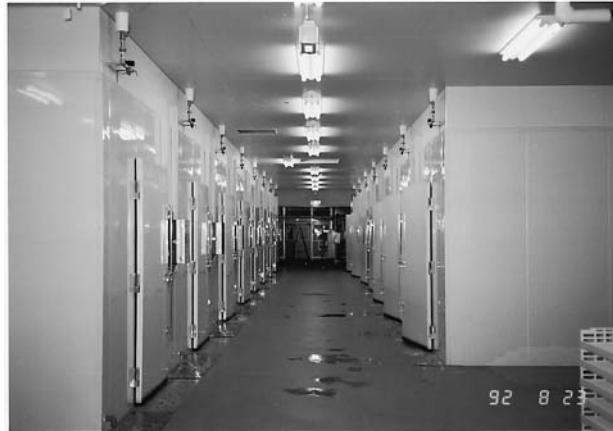
Figure 19 Automatic control fermenter. (Courtesy of Suzuyo Kogyo Co. Ltd.)
