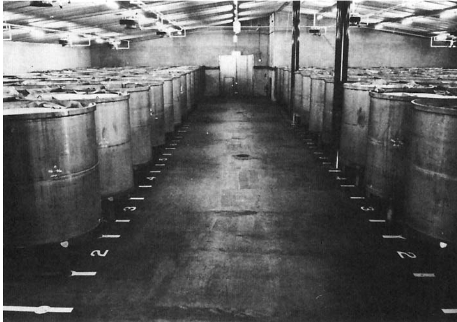
Figure 10 Fermenting room. (From Ref. 10.)
